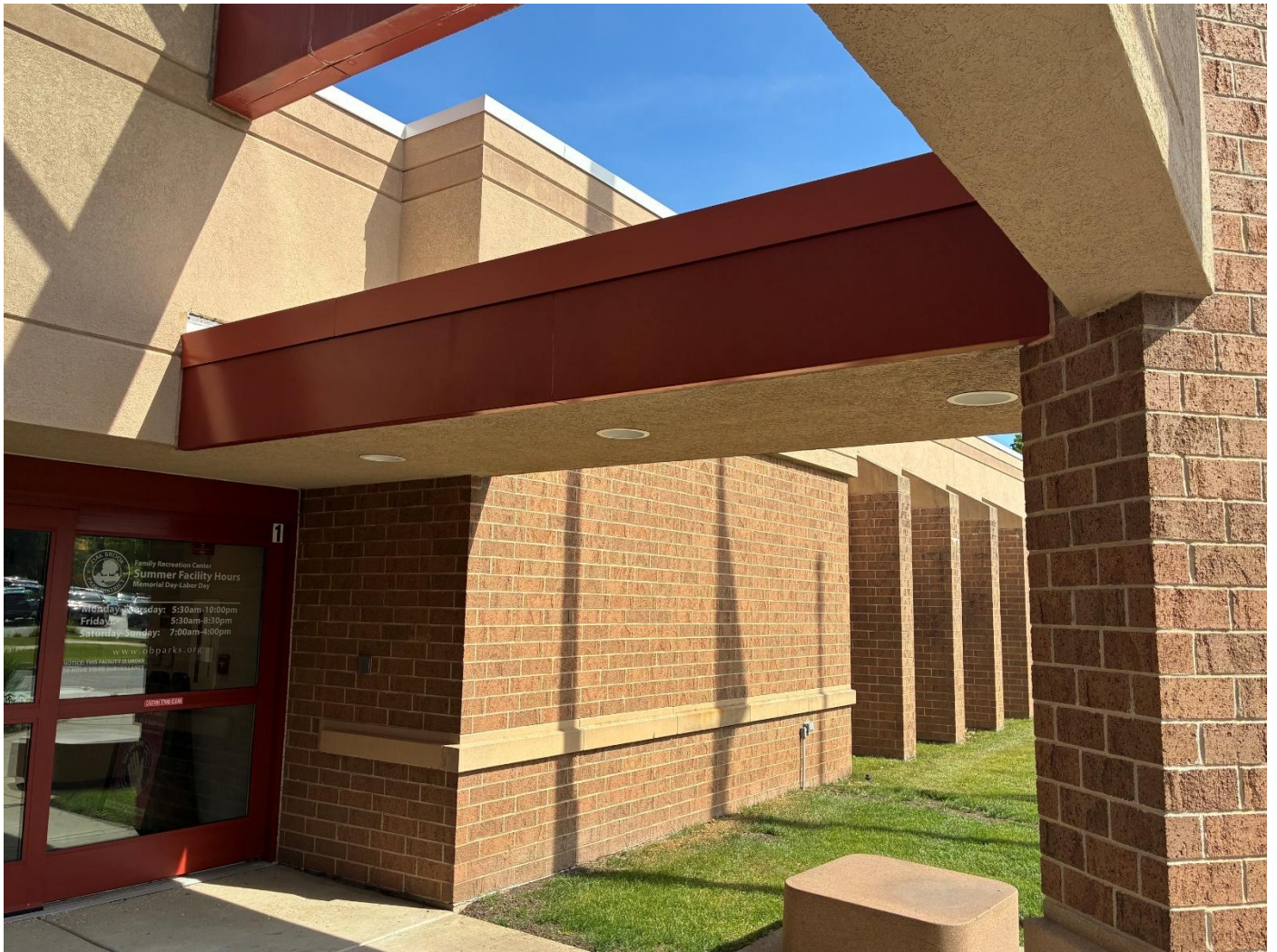
Awning Ceiling and trim.
