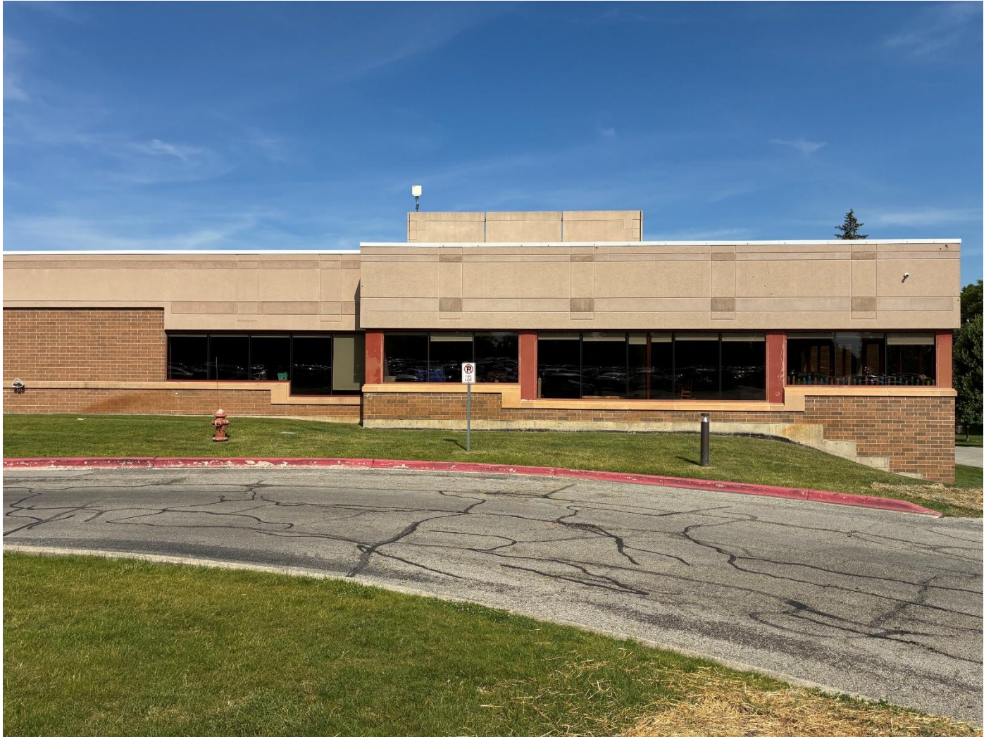
EIFS painting/repairs and window trim.
