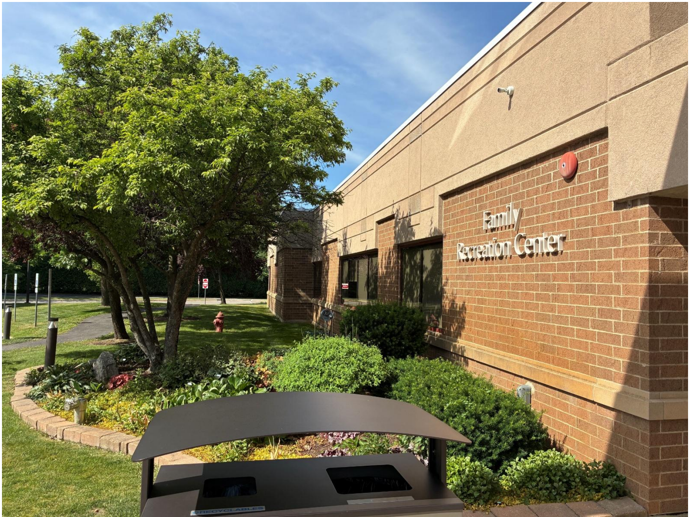
EIFS painting/repairs and window trim.
