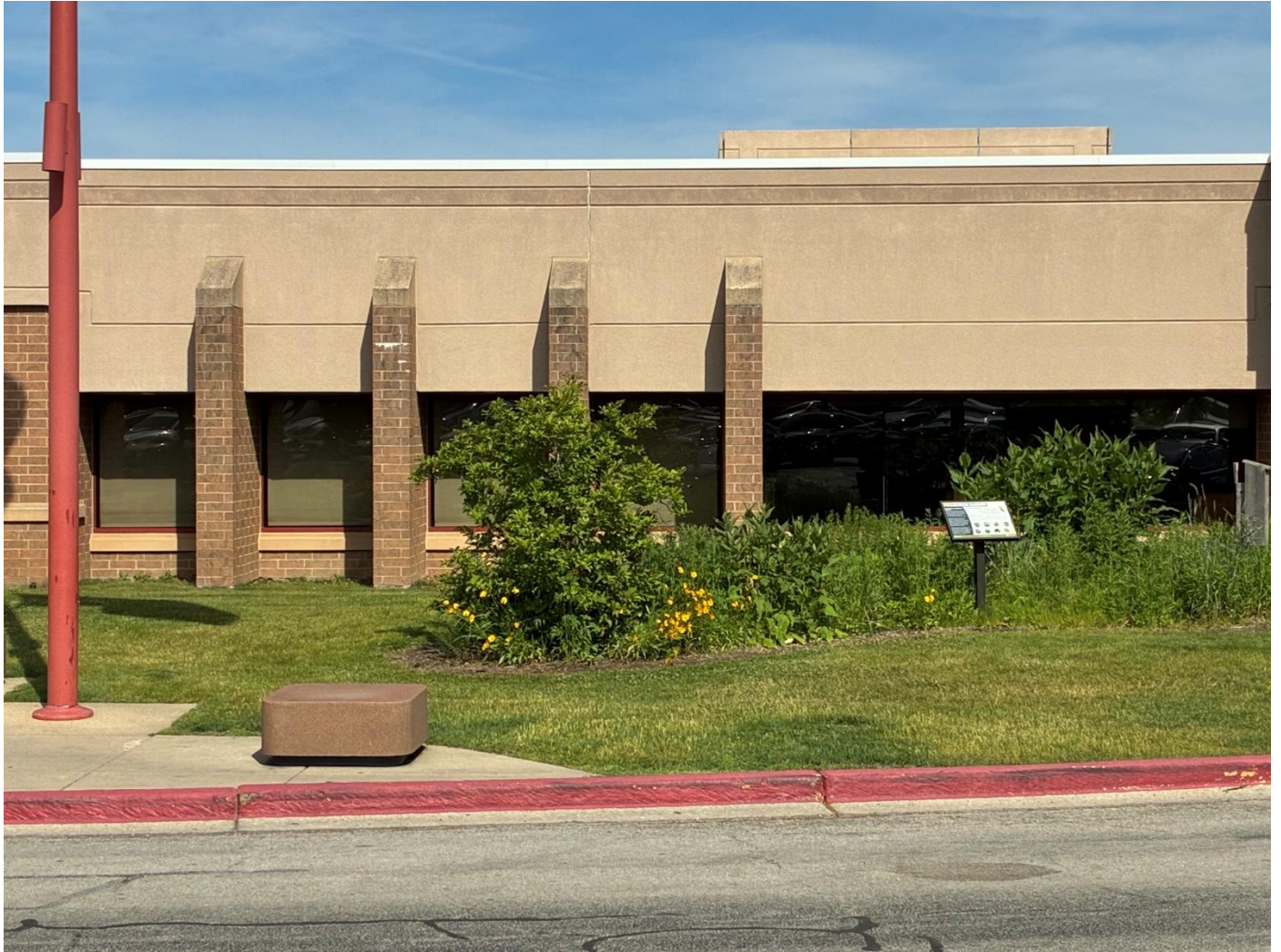
EIFS painting/repairs and window trim.
