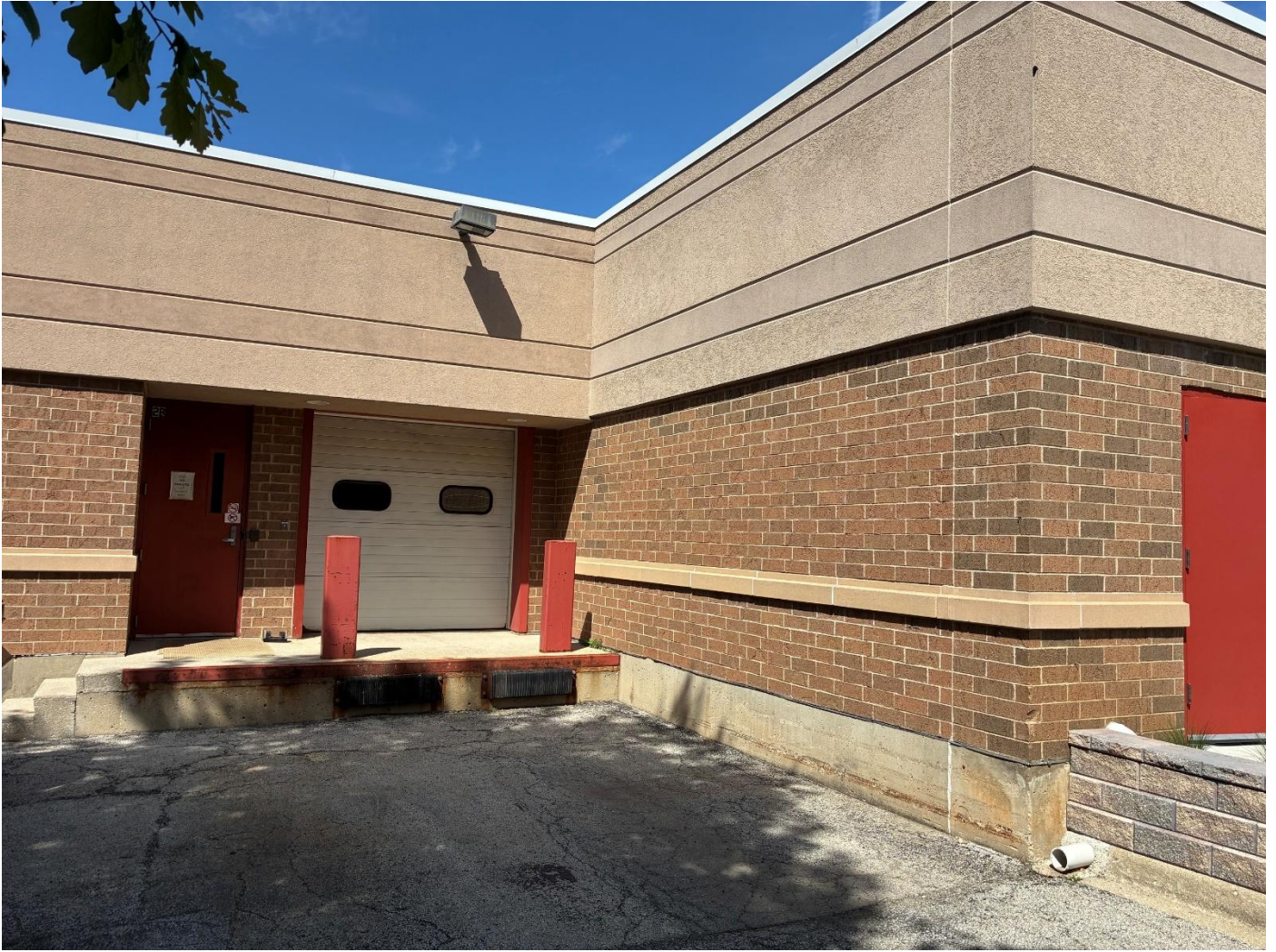
EIFS painting/ repair, door (#2B), garage door trim, two bollards, and truck stop.
