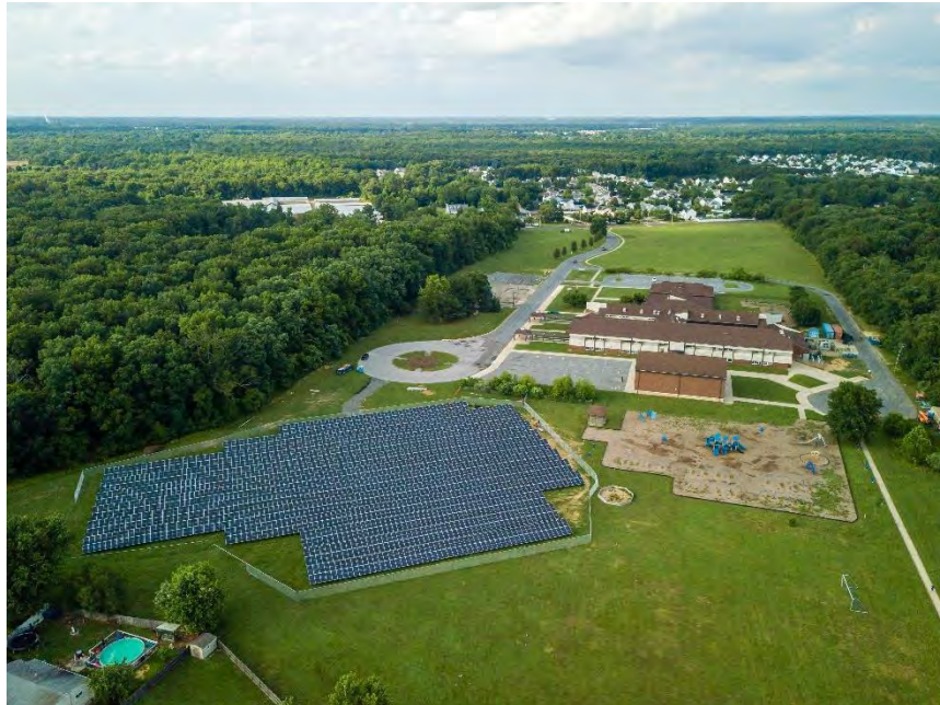
Figure 9. 840 kW Radix Elementary School – Township of Monroe
