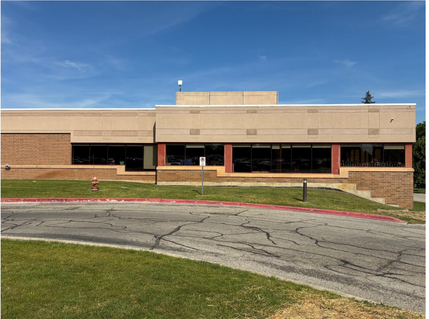
EIFS painting/repairs and window trim.
