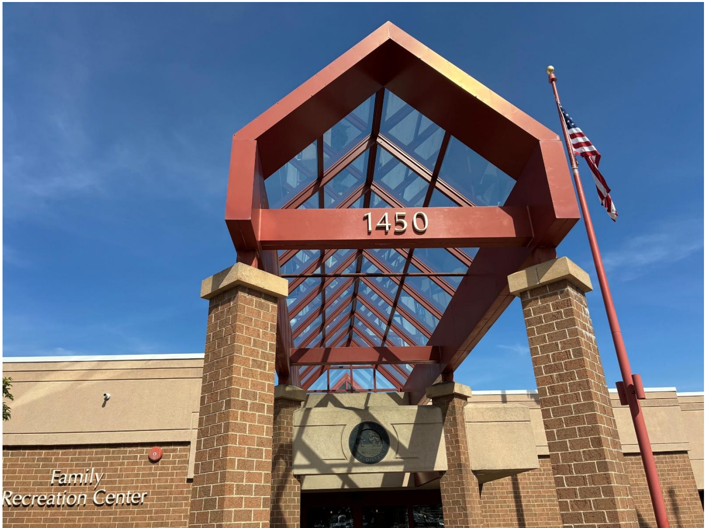
EIFS painting/repairs, Awning (both sides).
