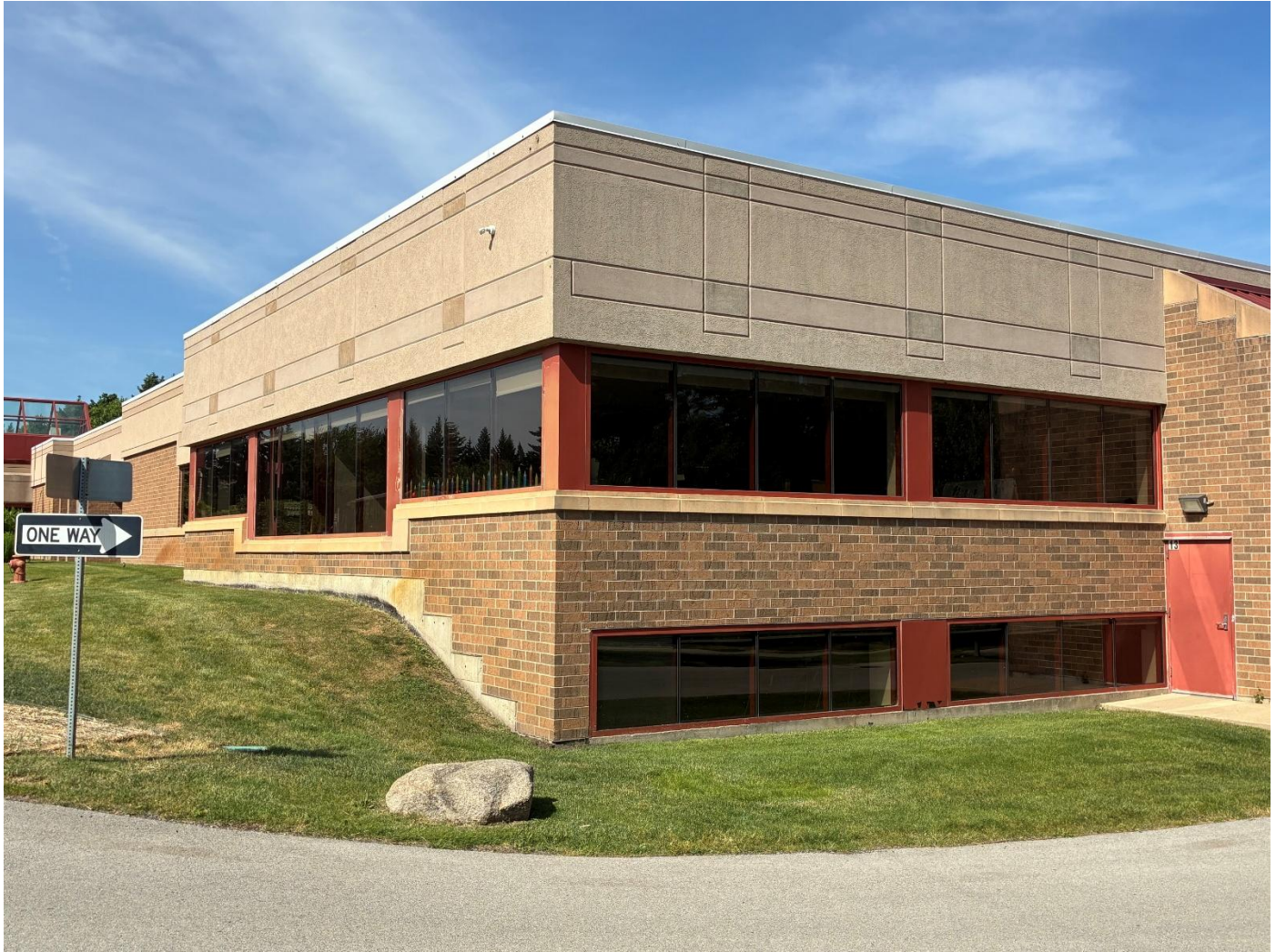
EIFS painting/repairs, Door (#13) and window trim.
