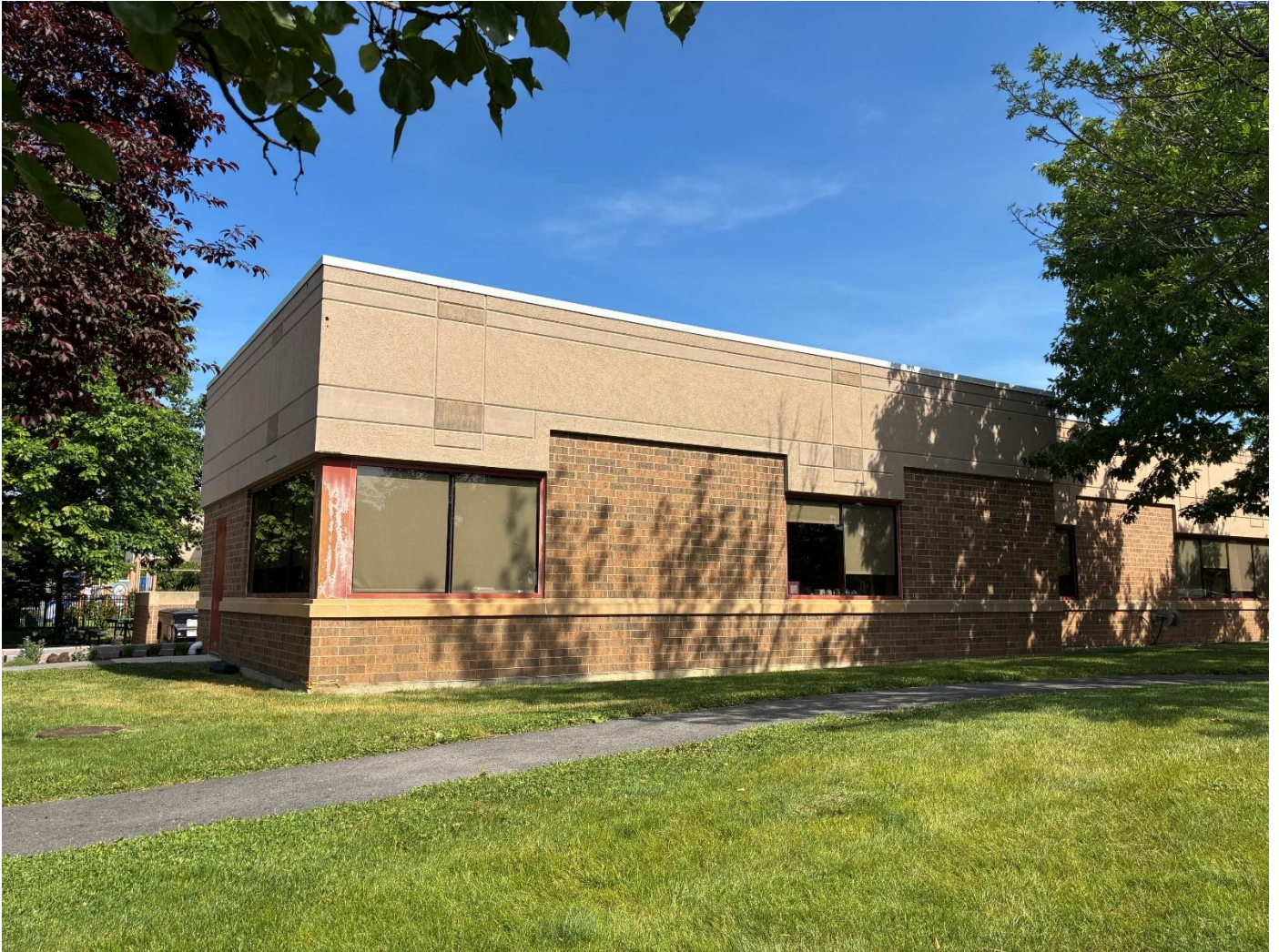
EIFS painting/repairs and window trim.
