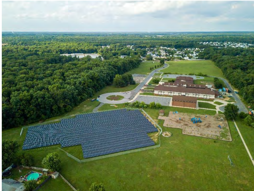
Figure 9. 840 kW Radix Elementary School – Township of Monroe
