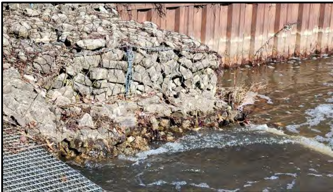
Photograph 7: Rock displacement, wire distortion and corrosion at gabion wall
