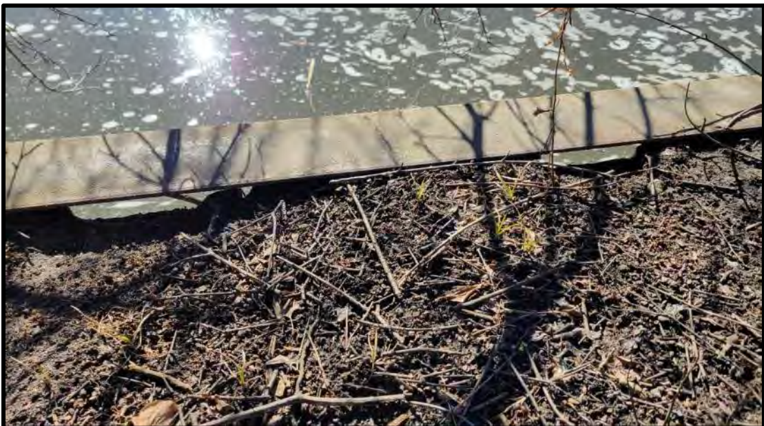
Photograph 14: Voids between the top plate and sheet piling
