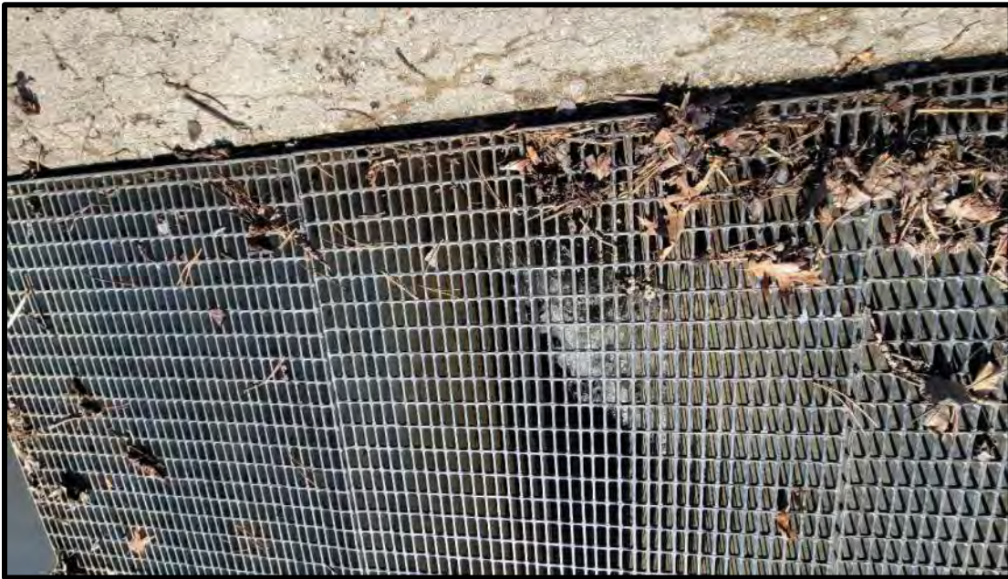
Photograph 18: Debris buildup on grate & water swirling at north footing
