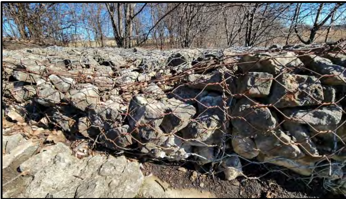
Photograph 6: Rock displacement, wire distortion and corrosion at gabion wall
