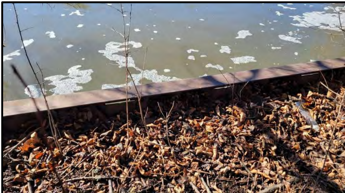
Photograph 15: Eroded backslope behind the sheet pile wall
