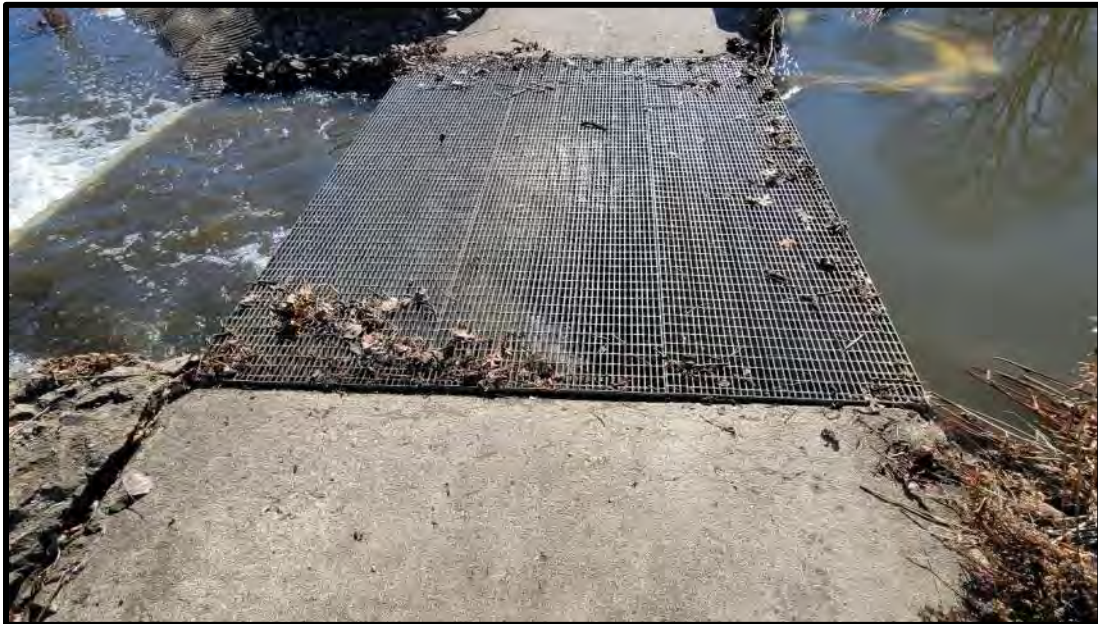
Photograph 2: Spider cracking in north approach slab & debris buildup on grate
