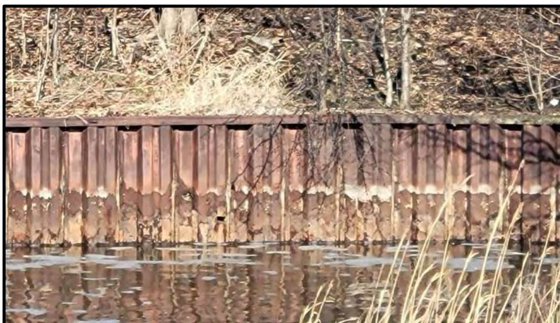
Photograph 12: Deterioration of steel sheet pile retaining wall
