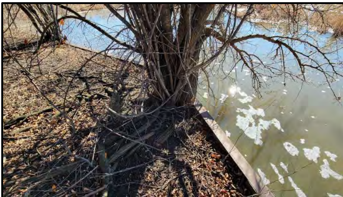
Photograph 16: Vegetative growth and slope erosion at the top of wall
