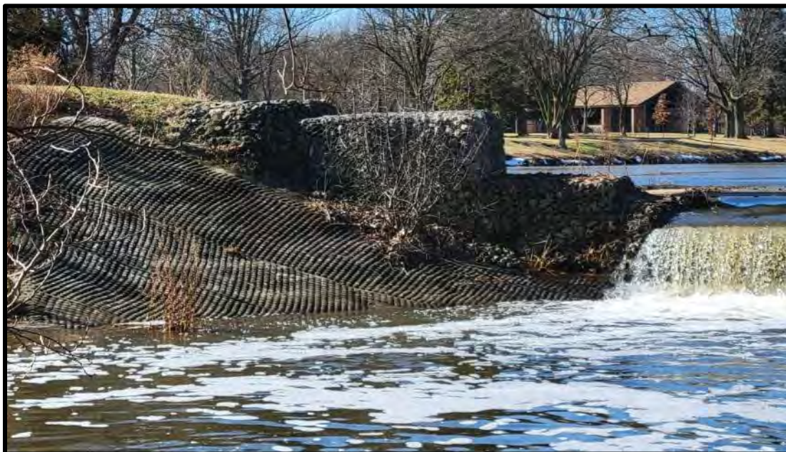
Photograph 19: CIP concrete mattress on downstream side of structure – Looking west
