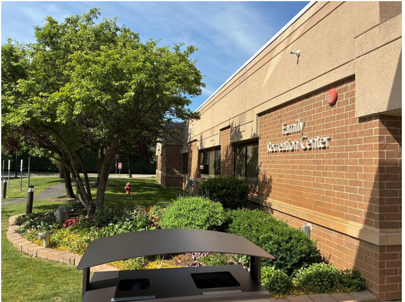
EIFS painting/repairs and window trim.
