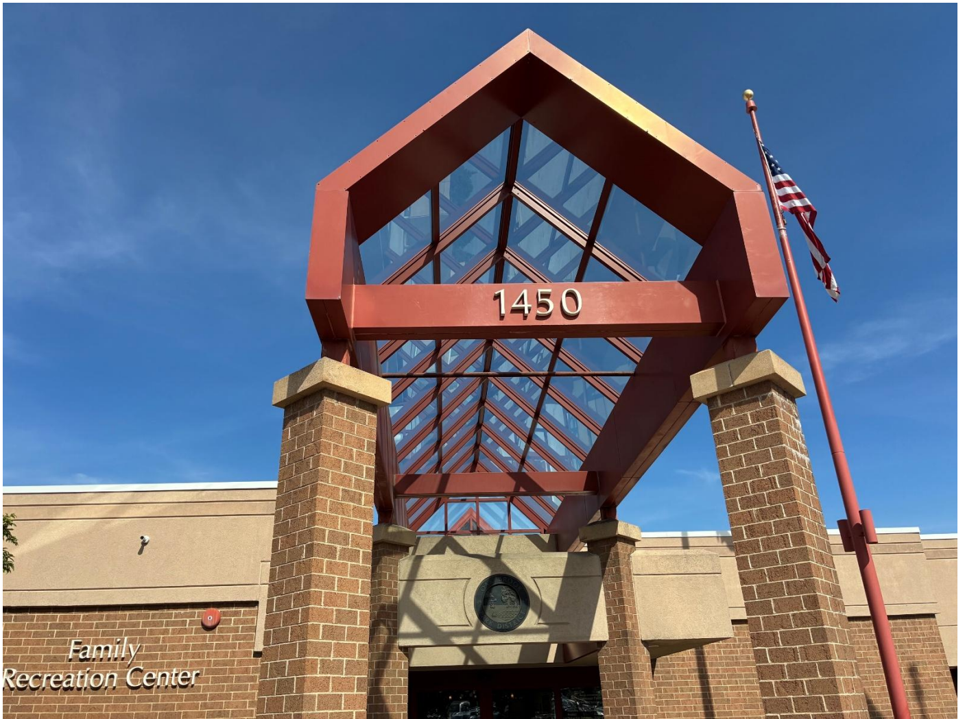
EIFS painting/repairs, Awning (both sides).
