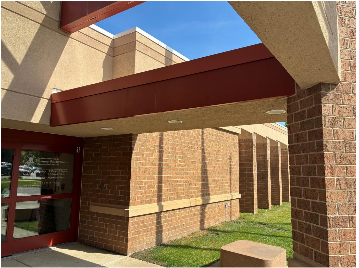
Awning Ceiling and trim.
