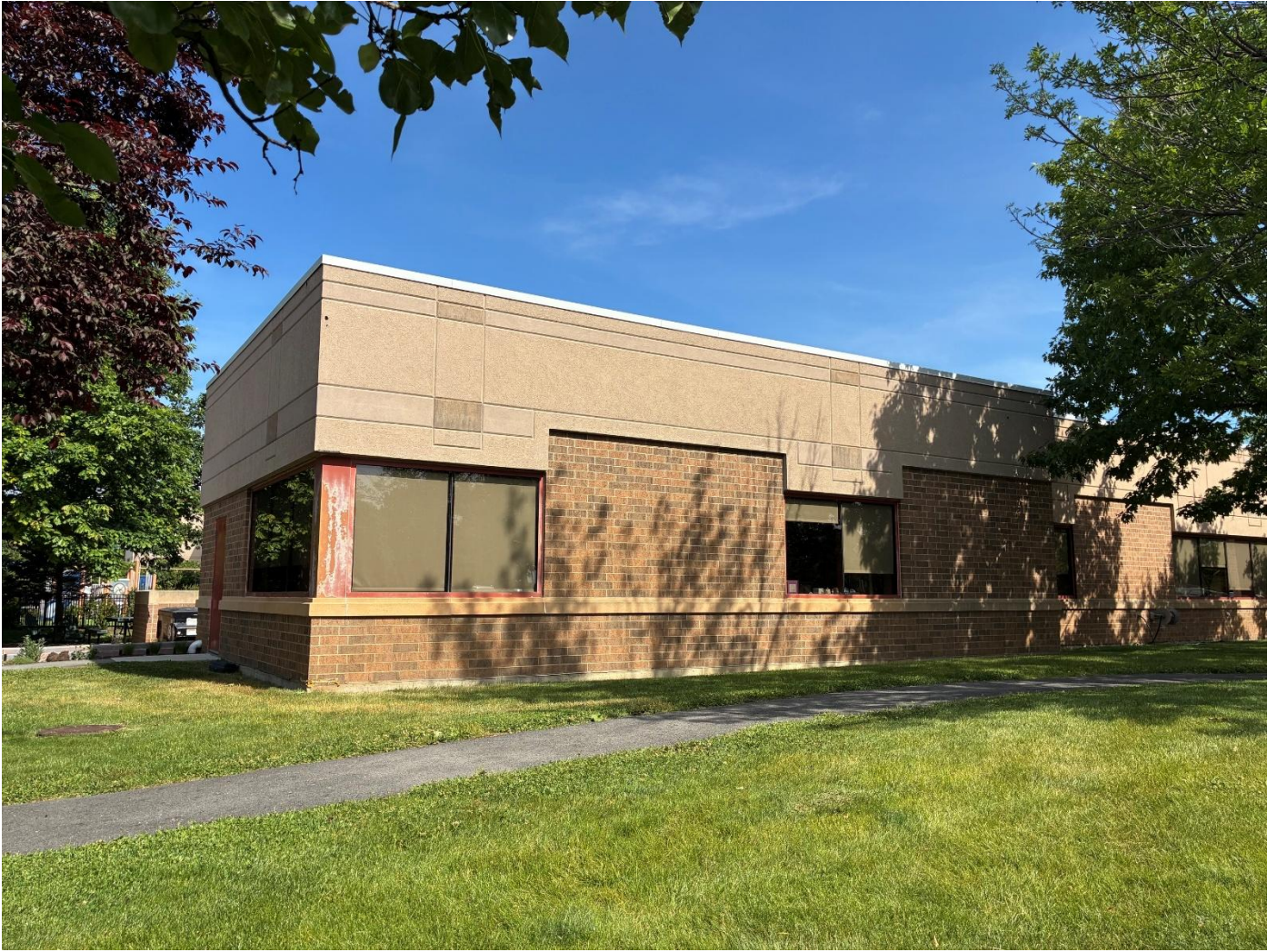
EIFS painting/repairs and window trim.
