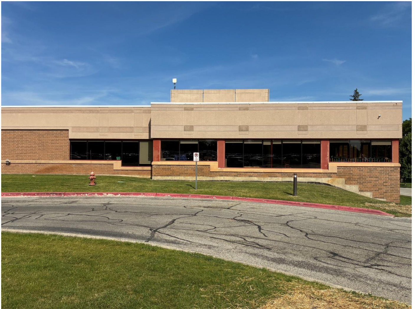
EIFS painting/repairs and window trim.
