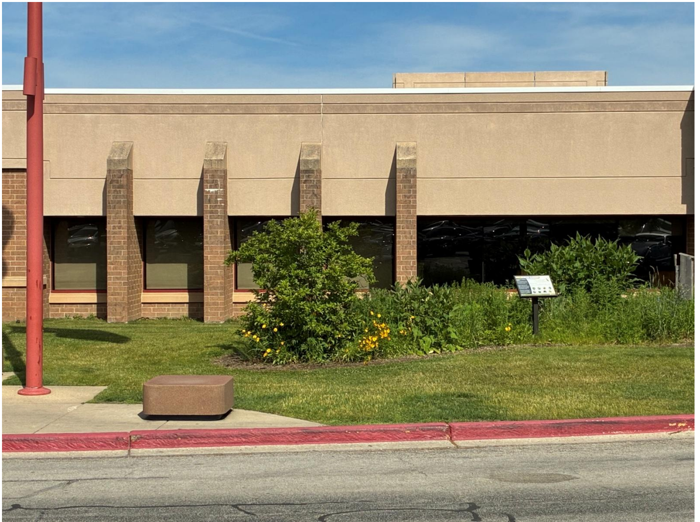
EIFS painting/repairs and window trim.
