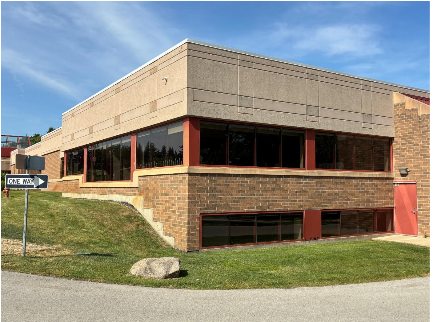
EIFS painting/repairs, Door (#13) and window trim.
