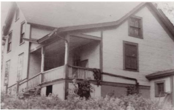
Farmhouse in 1939 before renovation
